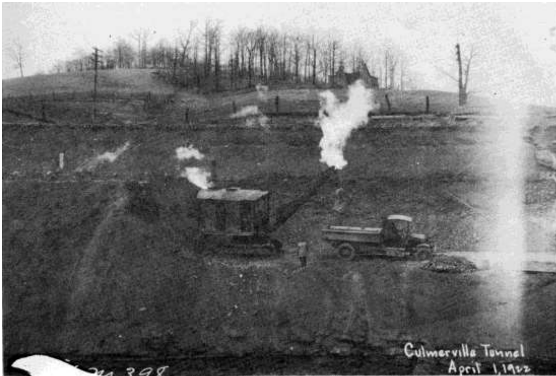
An ERIE steam shovel was used to help uncover the Culmerville tunnel in 1921 and 1922 Picture by B. & L.E. R.R.
