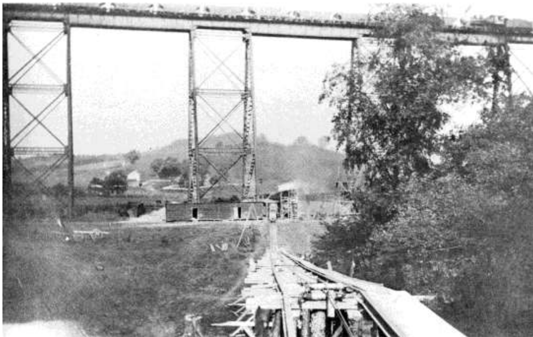
The original 139 foot high trestle that spanned the Bull Creek Valley at Culmerville. It was used from 1897 until 1912 when the present fill was completed. Picture from Bessemer and Lake Railroad
