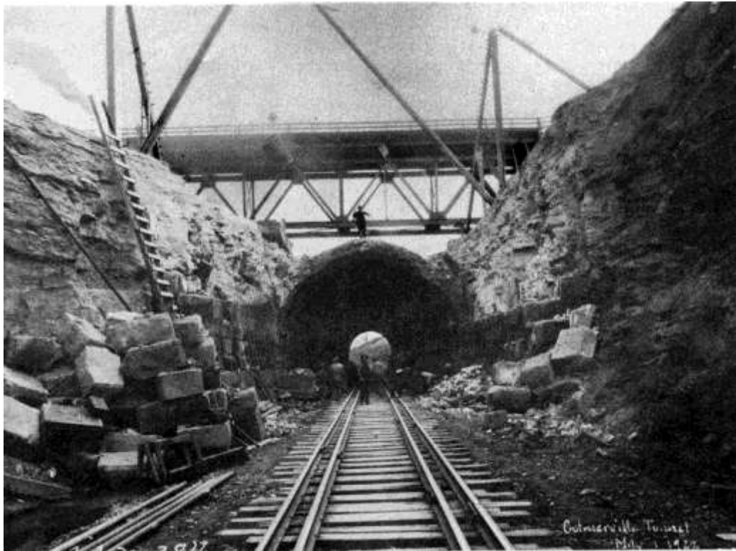
Drainage Problems in the tunnel and the use of larger locomotives required the removal of the tunnel. This 1922 picture shows the bridge almost completed and the tunnel work well underway. Photo from B. & L.E.R.R.
