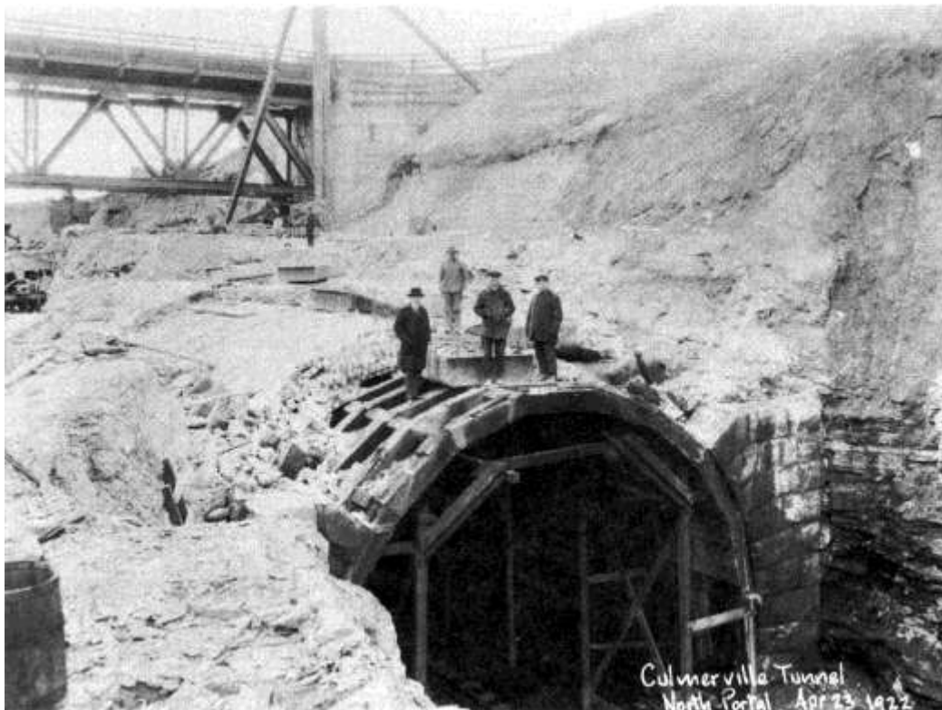
The wood construction inside the tunnel was bracing used to shore the tunnel when it started to cave in. This did not eliminate the problem. Picture by B. & L.E. R.R.
